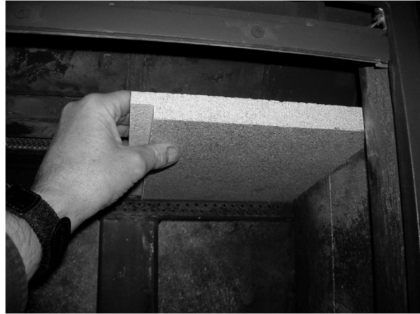
Figure 19 (cont.) - Removing/Replacing the Baffle for Inspection
