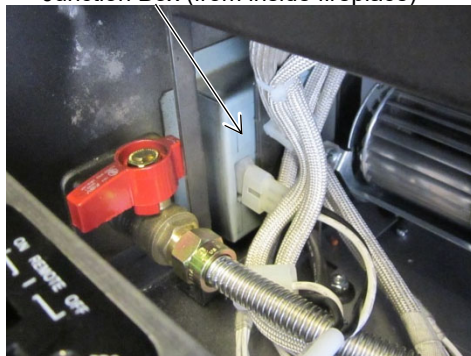
Junction Box (from inside fireplace)
