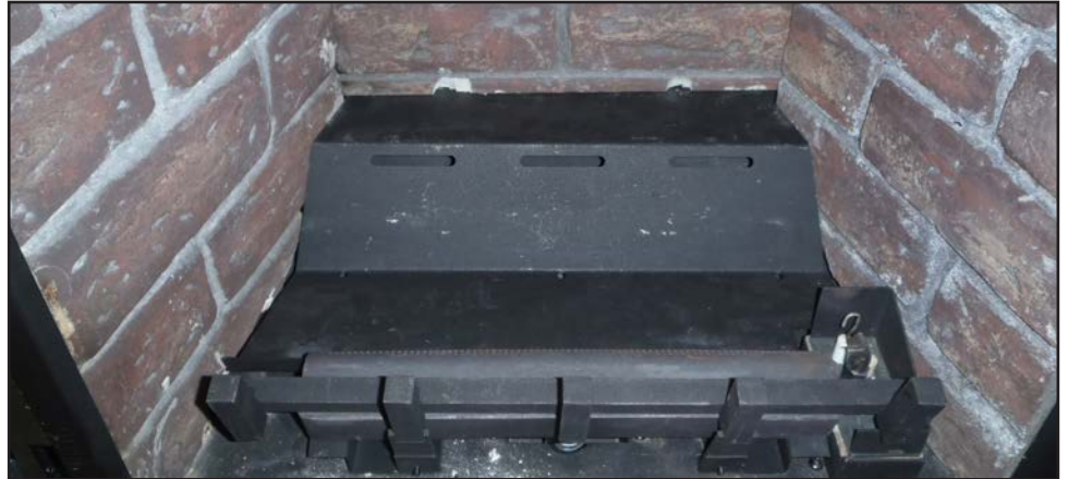
Figure 50. Empty firebox with grate and locator pins.
