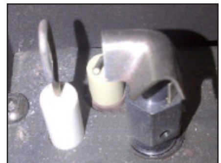
Figure 13: Proper Pilot Position
