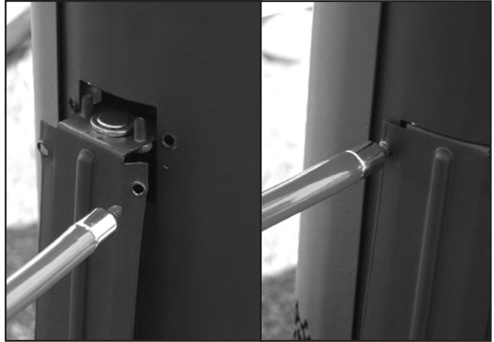
Figure 35: Spill switch installation.
