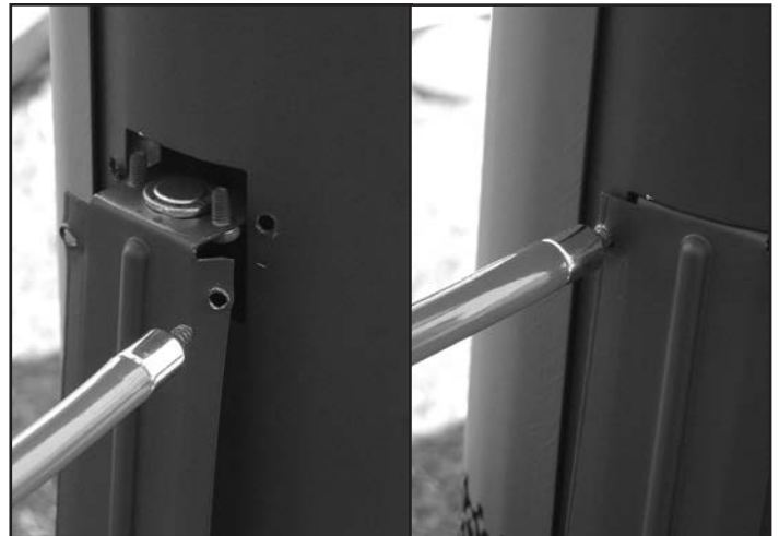
Figure 47: Spill switch installation.
